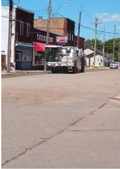
Day 1 Reclaiming the asphalt.
