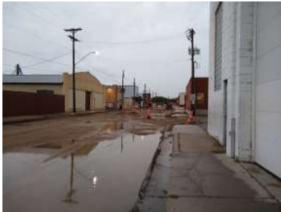
Day 5 Millings removed.
